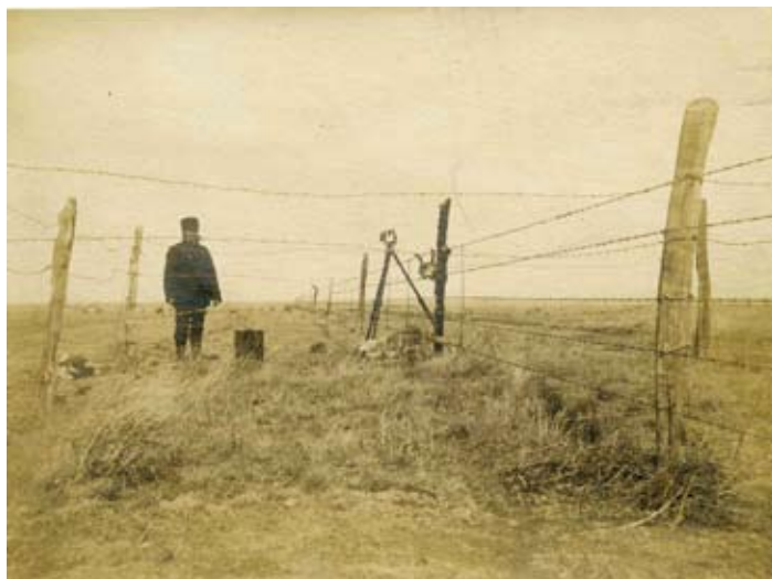
W. D. Twichell surveying the 103rd meridian between Texas and New Mexico, 1903. Note the box to Twichell’s side containing his surveying equipment, and the solar compass on a tripod that stands over the surveying monument (piled rocks) being documented by the photo. A closer look reveals a stack of wolf hides on the ground and an antelope skull on the fencepost.
